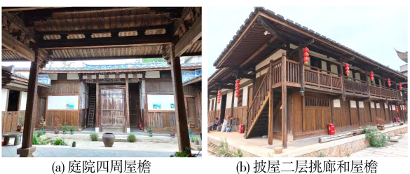
图 11 古厝内外屋檐遮阳结构 Fig.11 Sunshade structure of the ancient house eaves
