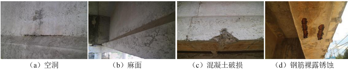
图 1 钢筋混凝土梁常见病害 Fig.1 Common diseases of concrete beams
