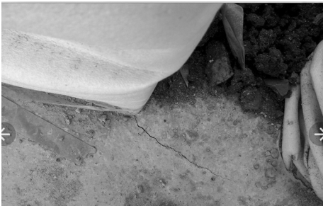
图 6 冠梁裂缝 Fig.6 Diagonal crack of top beam
